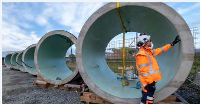
Pipes from Hynds ready for laying
