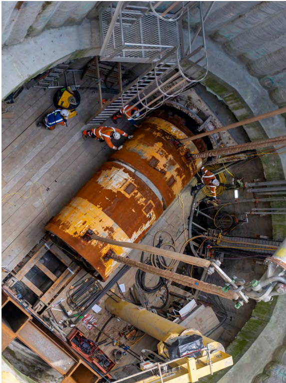
Lowering the mTBM at Miranda
