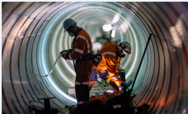
Welding work in the link sewer
